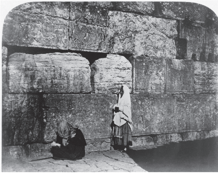
“Exterior of Haram-Ash-Sharif, Wailing Place of the Jews” by Peter Bergheim (1865). The newly available photo allows us to explore details usually not seen before, such as the Hebrew memorial notices written on the Wall. Bergheim established a photographic studio in the Christian Quarter of the Old City of Jerusalem. A converted Jew, he was well aware of Jerusalem’s holy sites. 8
